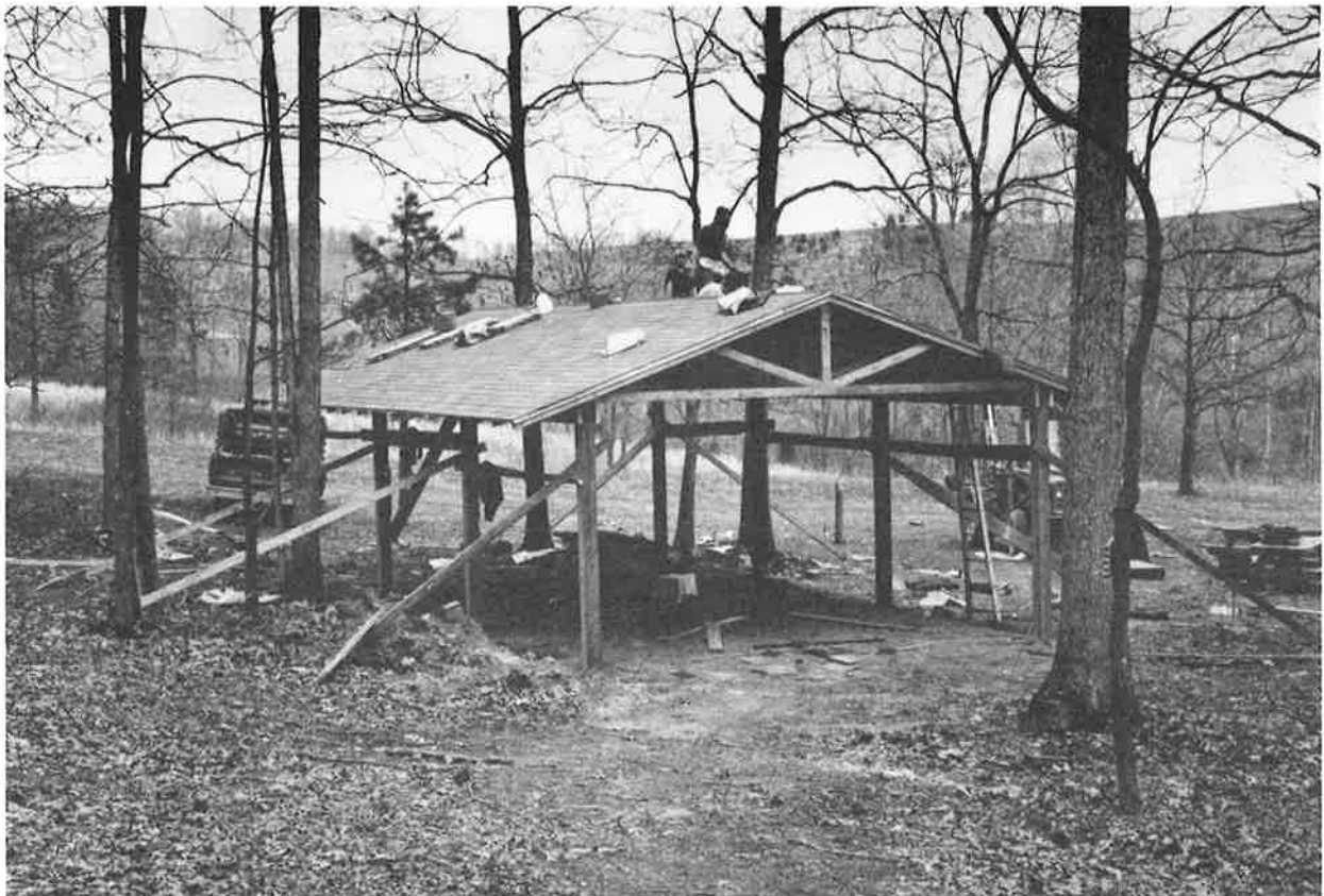
SHELTER AT LEDGES BEING BUILT
