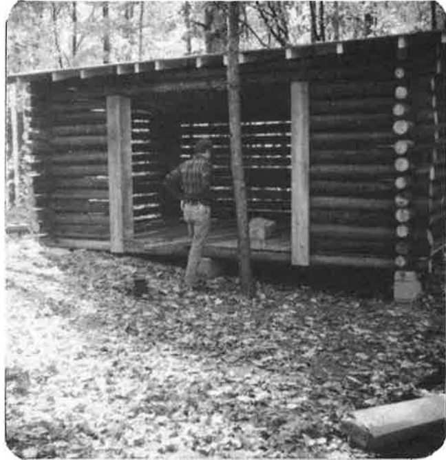
ADIRONDAKS BEING BUILT
